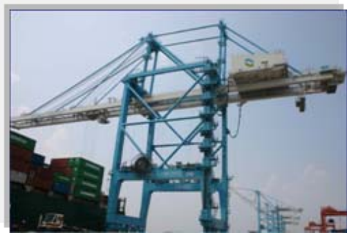
Elevating Girder Crane (ZPMC)
