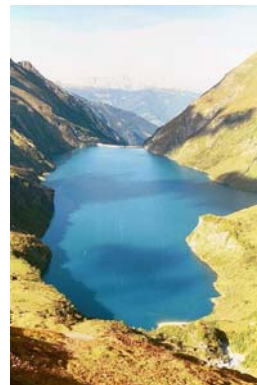
Kaprun, Reservoir Mooserboden view, Austria A water Power Plant in Salzburg.
