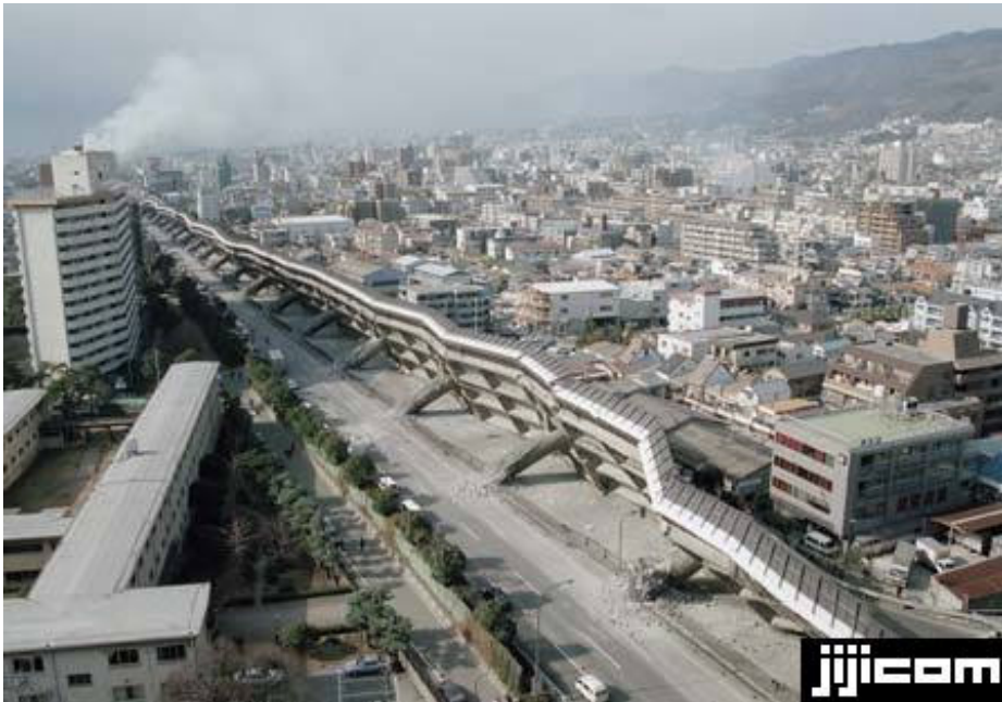
Hanshin-Awaji Great Earthquake Disaster Jan. 17, 1995. M 6.7 (Photo: Jiji com.)
